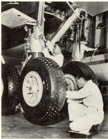
Mechanics go over the anti-skid tires and check the new boom installation prior to flight test.
